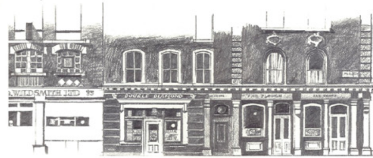
LITTLE RUSSELL STREET, NORTH SIDE
