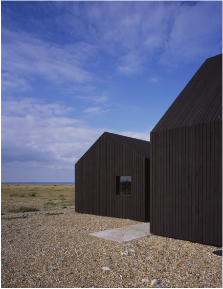
Above: Black stained timber cladding, shingled ground Right: Kitchen window, South elevation
