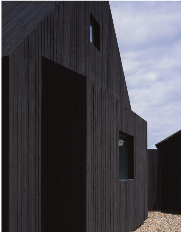
Black stained timber cladding
