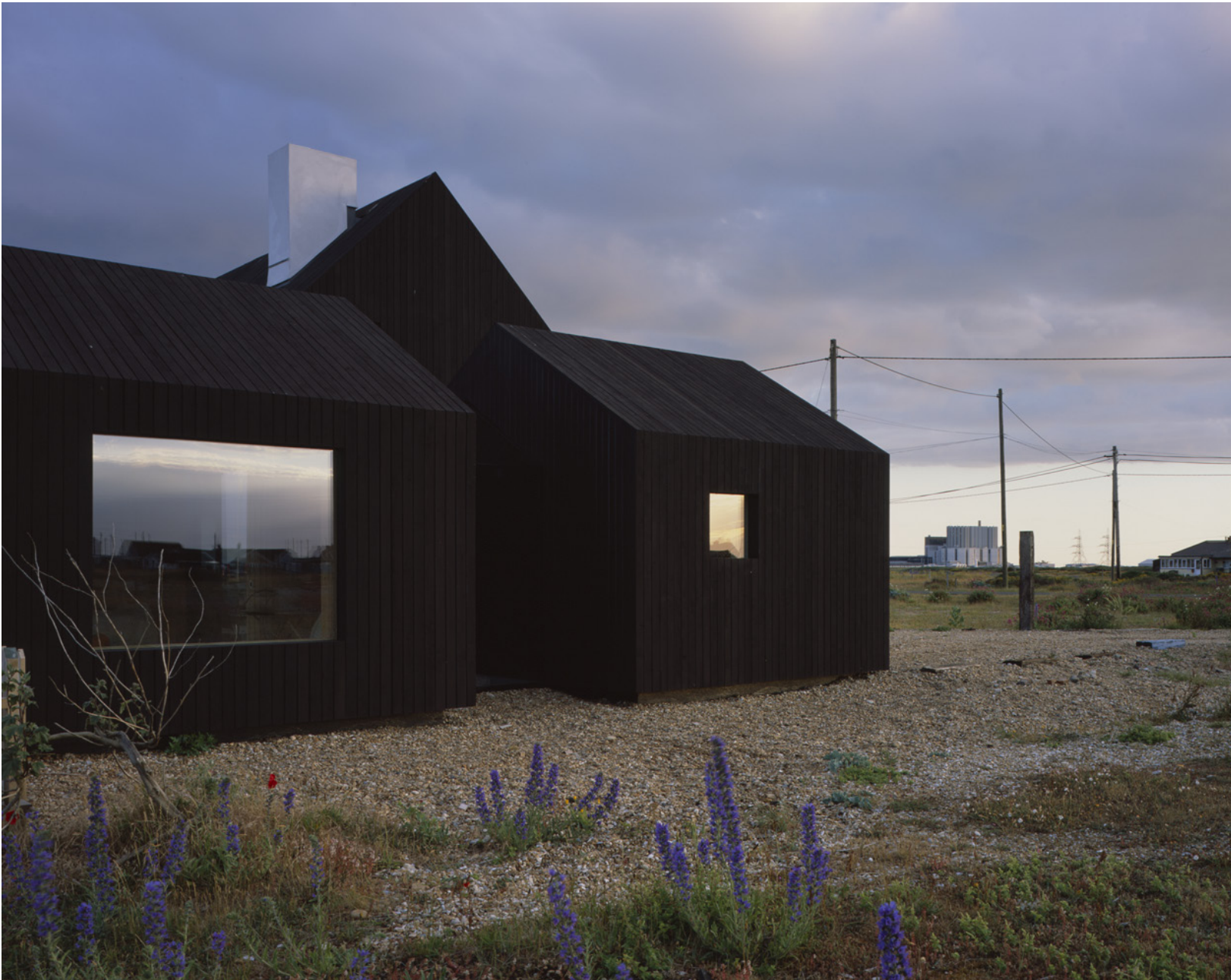
Power station, dusk
