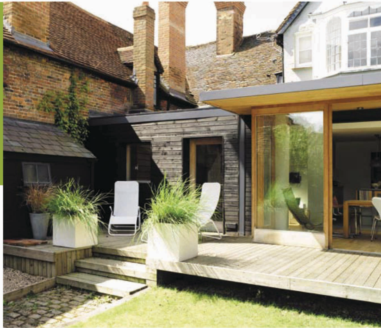
Right: A large deck leading from the dining area outside allows the interior and exterior of the extension to be used as one
